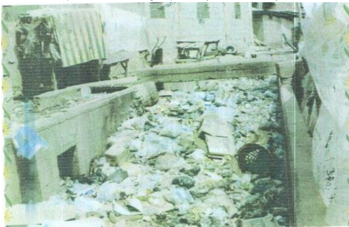
Figure 4: Refuse-choked concrete-channelized segments of River Ajilosun at Agere in Oja Oba, Ado-Ekiti.
