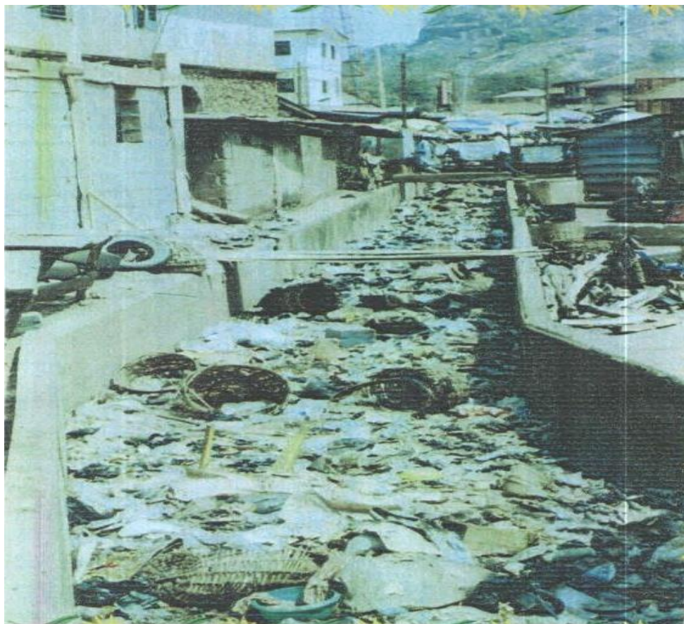
Figure 3: Refuse-clogged section of River Ajilosun channel at Odo-Otu tributary of the river. The picture was taken during the peak of dry season in February, 2018.
