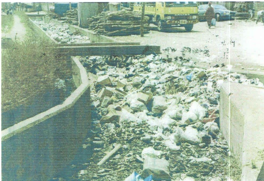
Figure 3: Refuse-blocked section of River Ajilosun channel at Atikankan in Ado Ekiti.
